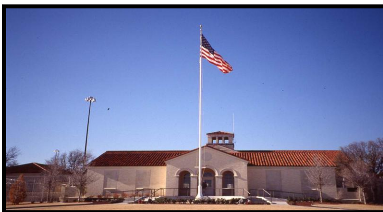
Entrance to Facility
